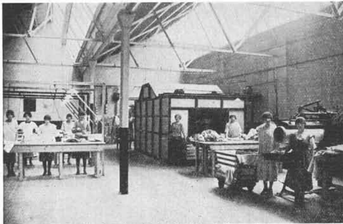
The Laundry. Drying Machine in the centre.
