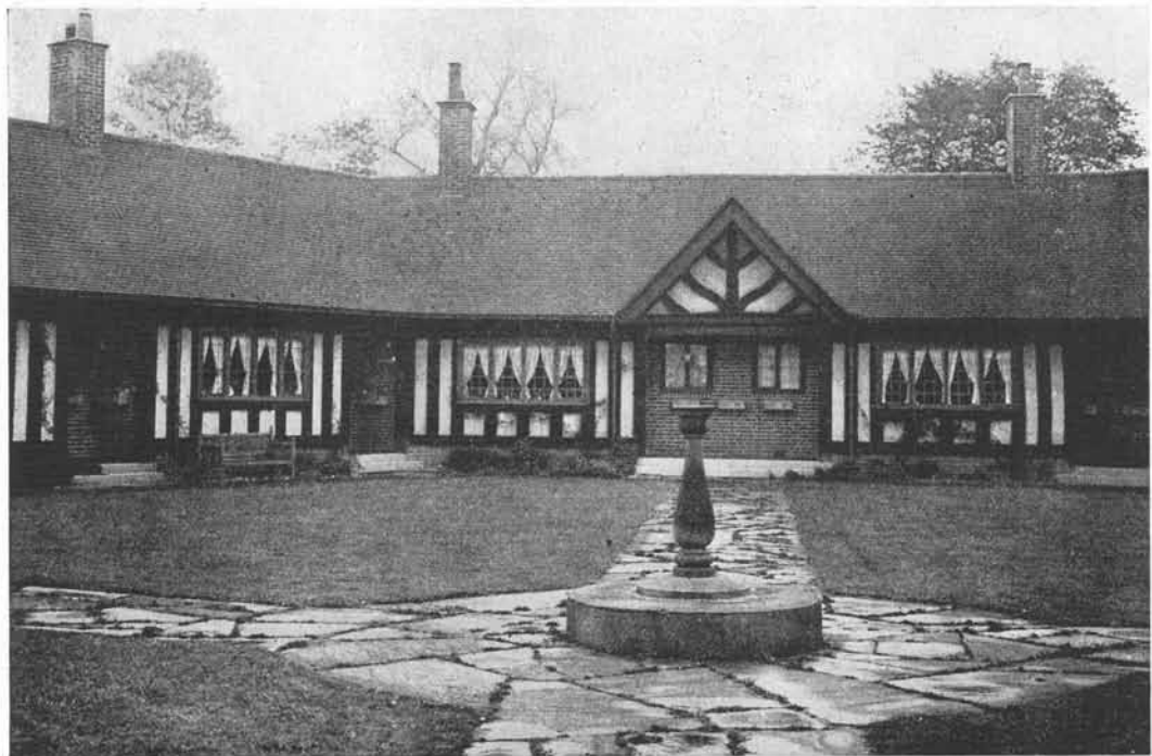
Portion of block of eight Almshouses, the gift of Miss Juliet Reckitt, in the Garden Village.
